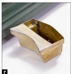
To take care of gaps, Rick squeezes the joint closed, then heats it to liquefy the solder.
