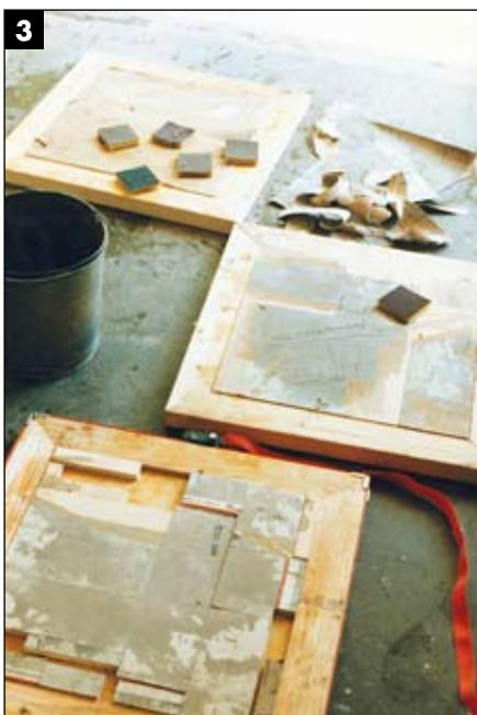
**To remove drywall's paper covering, soak the paper with water. Use sandpaper on the last stubborn bits of paper.**
