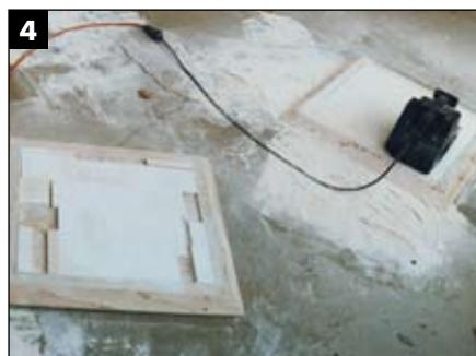
**Notice how the frames' sides have been sloped at 45 degrees. A belt sander quickly levels the drywall surface but also makes one whale of a mess; wear an industrial-grade respirator and eye protection.**
